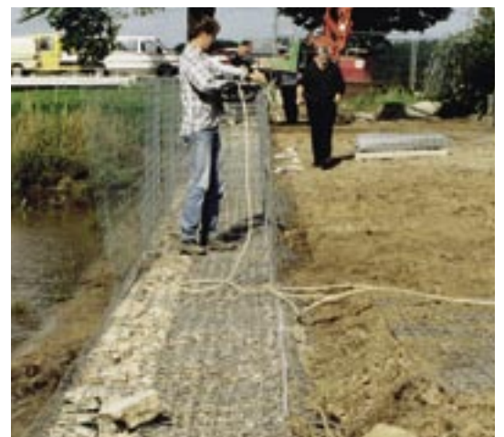
September 2001, detail systeem 'Terra+Wire+Mesh' ® gewapende grond.
